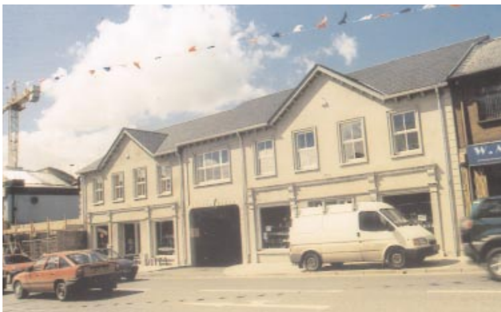
Before and after photographs of a UDP project in Market Street, Omagh.
